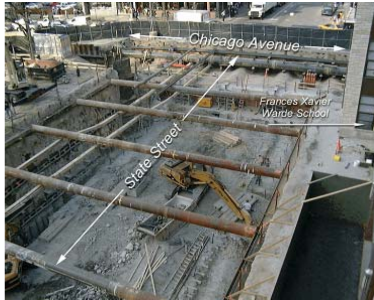
Figure 3.11 - Excavation Site (View from Roof of adjacent School) (After Bryson, 2002).
